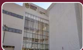
Hospital General "Tláhuac" CDMX
